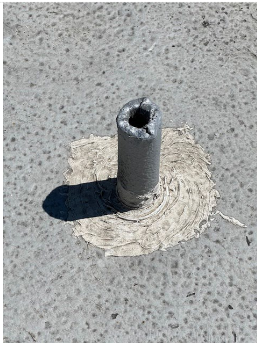
White Penetration -Lead Roof Jack
